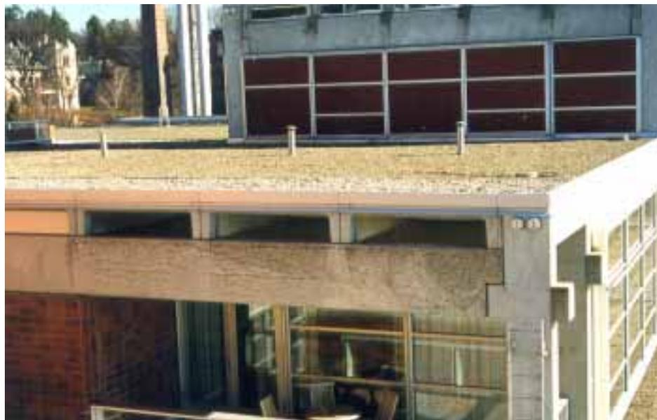
Fig. 10 The Norwegian Veritas House with prefabricated beams and columns. Note the cracked beams in the front
