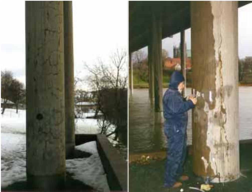
Fig.4: Map cracking and vertical cracks in columns of Elgeseter bridge. Note that the column (right photo) is wet of rainwater on western face (near the man) and dry on eastern face.
